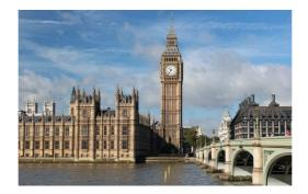
The bottom 200 feet of the tower's structure consists of brickwork with sand coloured Anston limestone cladding. The remainder of the tower's height is a framed spire of cast iron. The tower is founded on a 50 feet square raft, made of 10 feet thick concrete, at a depth of 13 feet below ground level. The four clock dials are 180 feet above ground. The interior volume of the tower is 164,200 cubic feet.
